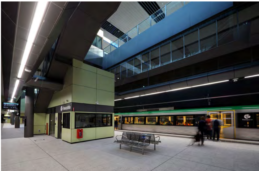
Figure 46 Redcliffe Station on Transperth's new Airport Line
