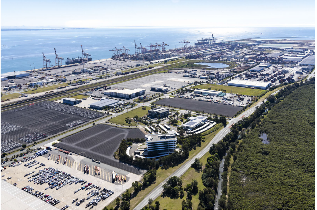
Aerial view over Fisherman Islands towards Brisbane Multimodal Terminal and the container wharves. Photo courtesy of Port of Brisbane Pty Ltd.
