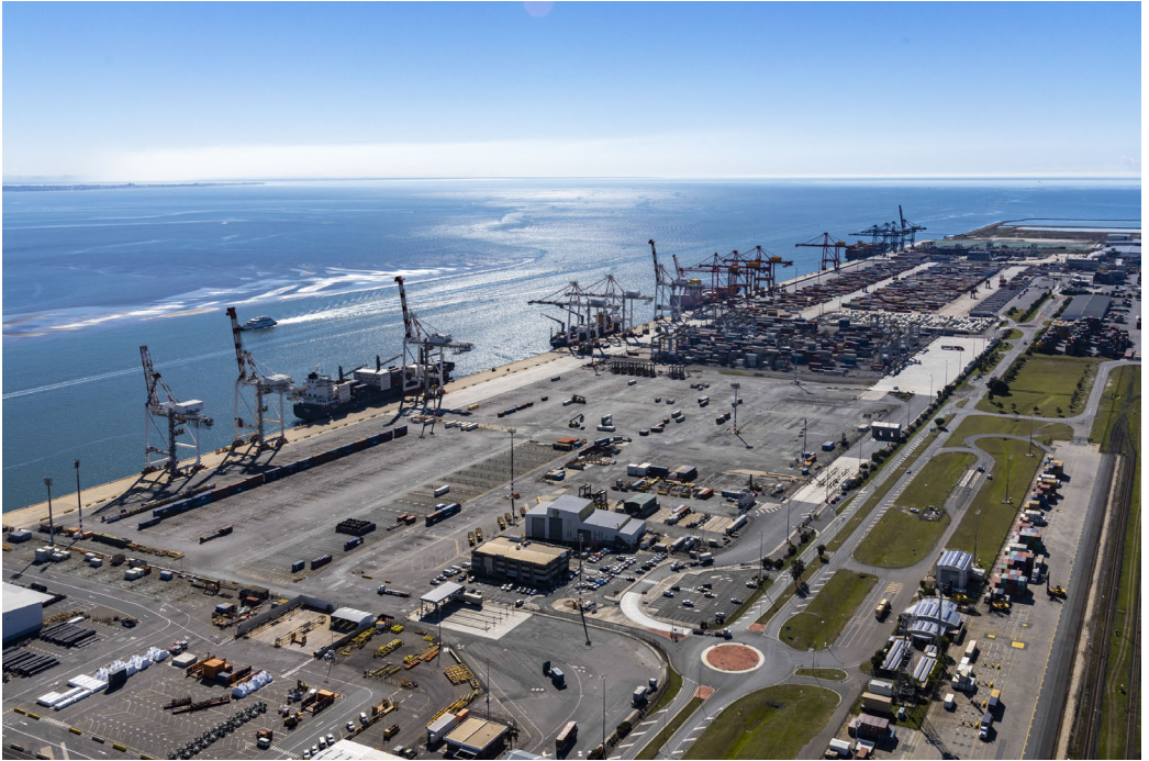
Port Drive and the Fisherman Islands container terminals. Foreground: DP World truck gates and Brisbane Multimodal Terminal. Photo courtesy of Port of Brisbane Pty Ltd.
