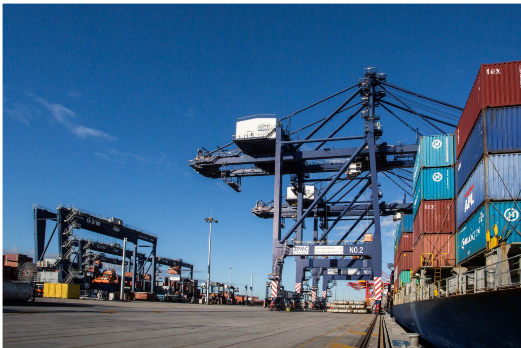
Vessel alongside at Brisbane Container Terminals. Photo courtesy of Port of Brisbane Pty Ltd..
