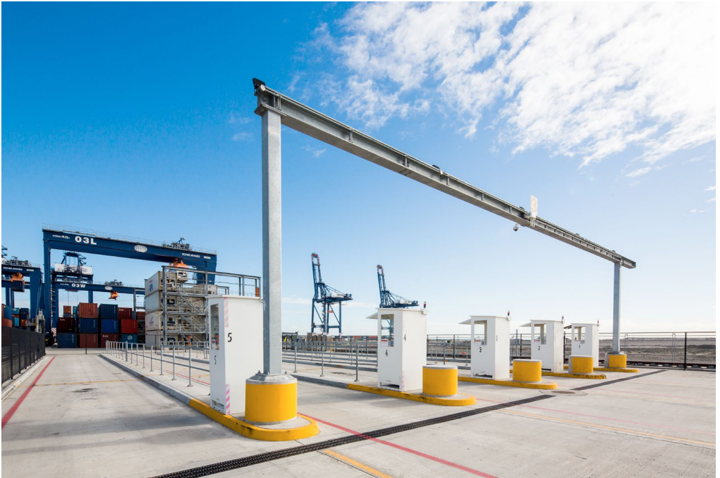
Truck loading area for automated straddle carrier; Brisbane Container Terminals. Photo courtesy of Port of Brisbane Pty Ltd.
