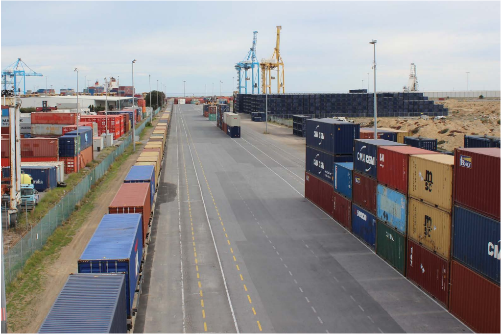
Rail siding, rail intermediate stacks and retainer stacks at Flinders Adelaide Container Terminal. Photo courtesy of Flinders Adelaide Container Terminal.
