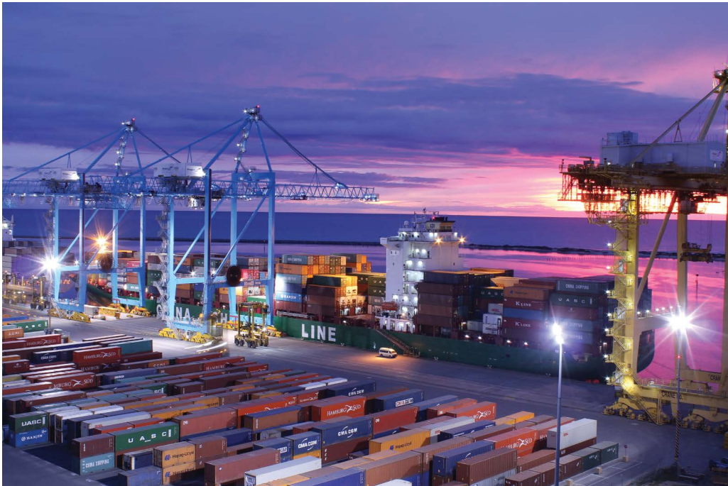
Two new cranes work a vessel at Flinders Adelaide Container Terminal. Photo courtesy of Flinders Adelaide Container Terminal
