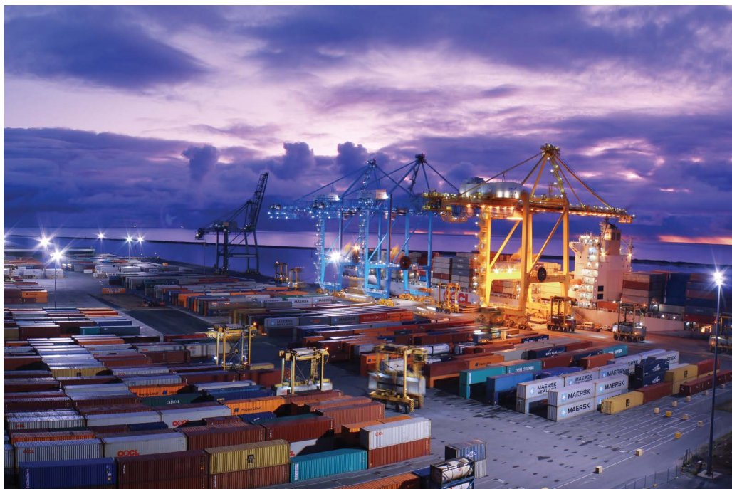
Two new blue post-Panamax Liebherr cranes were commissioned at the Flinders Adelaide Container Terminal in 2015. Photo courtesy of Flinders Adelaide Container Terminal.
